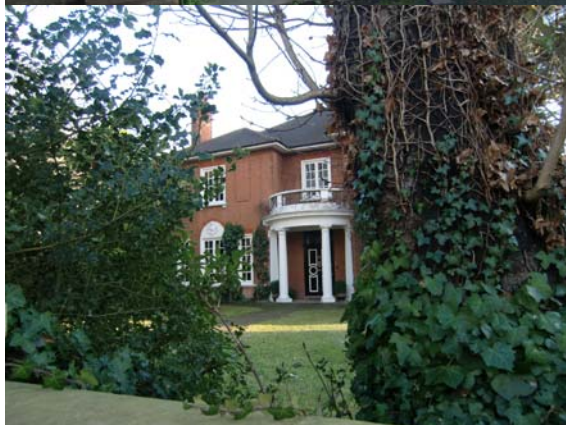
Locally listed 4 Roxborough Avenue
